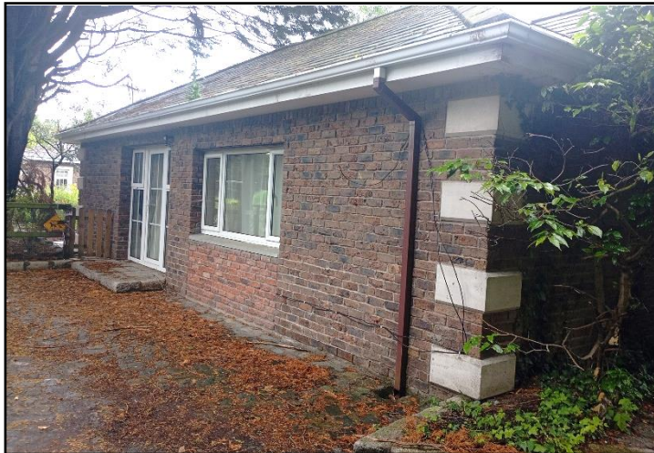
Plate 3: Existing building to be demolished (BL3)
