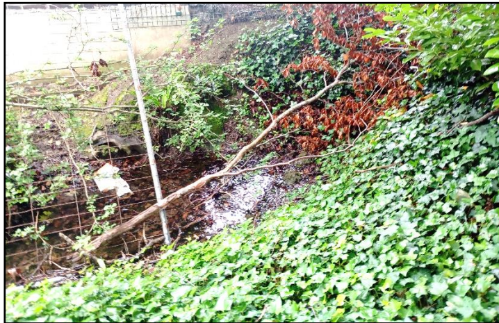
Plate 7: Drainage ditch to the west (FW4). To be infilled.
